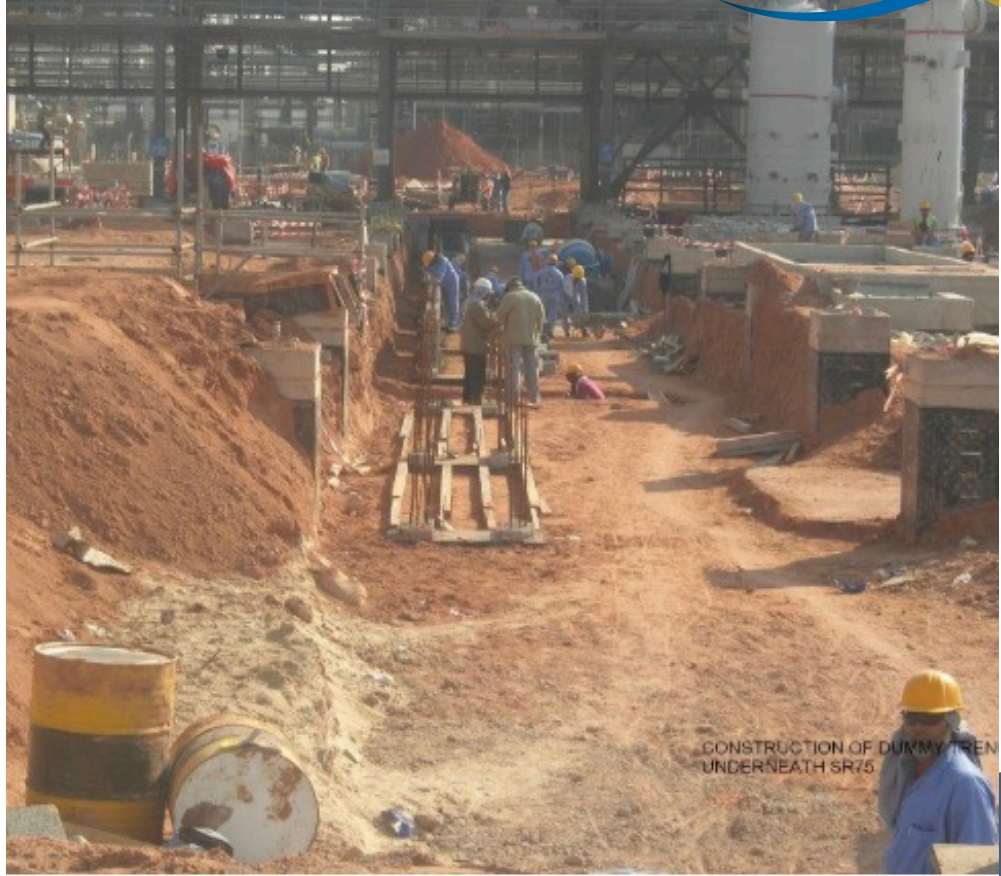
CONSTRUCTION OF DUMMY TRENCH UNDER SR75
